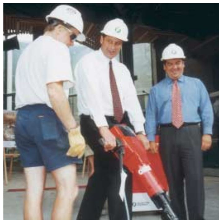
The Premier, Steve Bracks at the commencement of the renovation of the St Kilda Road building
